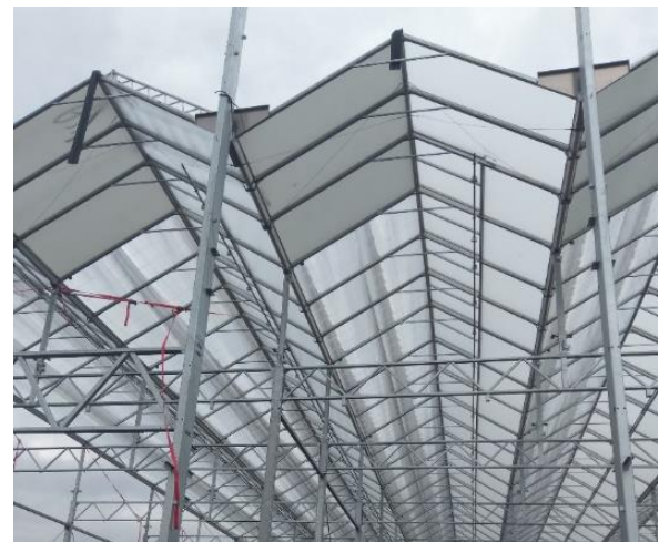
The first greenhouse under construction
